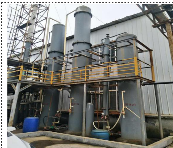
图 4-1 酸化釜废气一级二级碱喷淋
